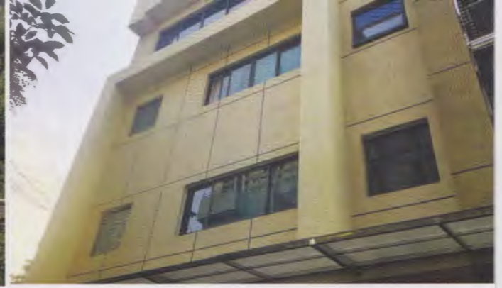
Building in Thailand using "G" brand glass
